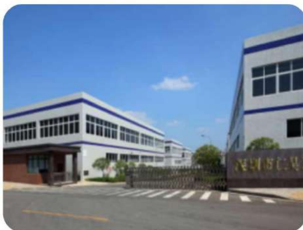
Renhotec(Shenzhen) Technology Ltd.,
